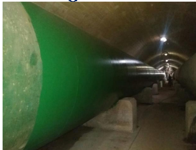
Pintura - Tubos de By Pass
